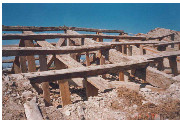
Total dismantling of the roof
