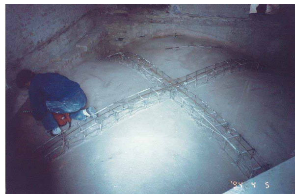
Specifics of the consolidation of the supporting vaults
