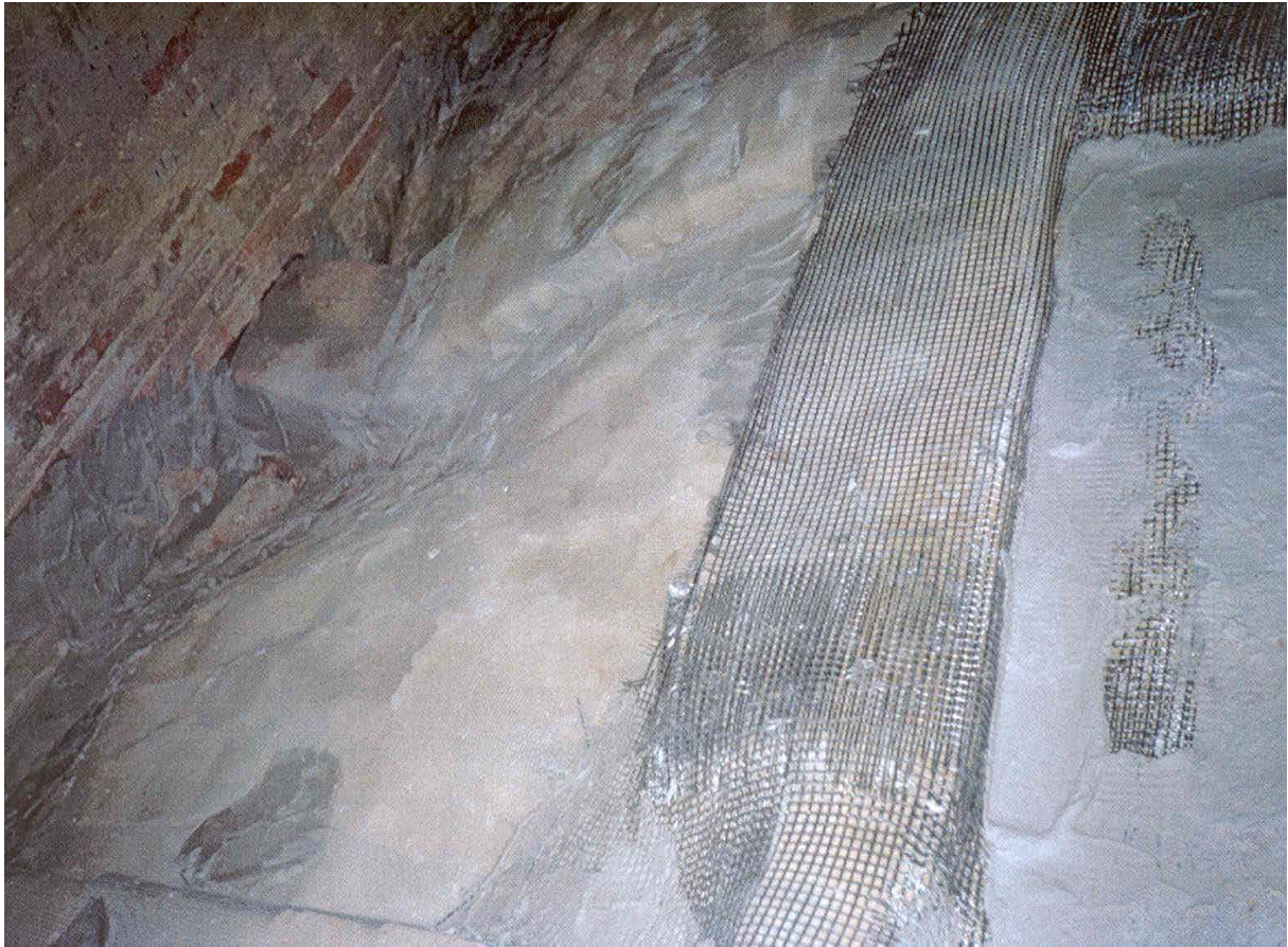
Restoration of the vault 3rd phase: reinforcement of the time with a fiberglass
