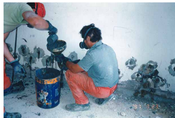
On the left execution of the chemical barrier against capillary rising moisture On the left the filling of the holes with special dehumidifying mortar
