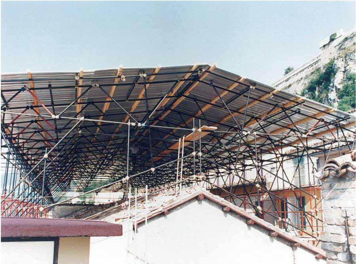
Provisional cover in pipes and joints
