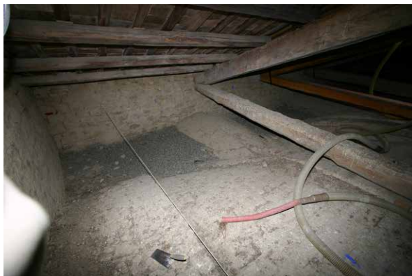
On the left particular consolidation of the under roof – On the right particular reinforcement of the under roof with a metal net
