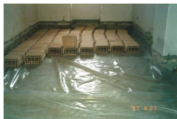
On the left the dismantling the floor for drainage – On the right laying of the nylon cloth and boards for drainage
