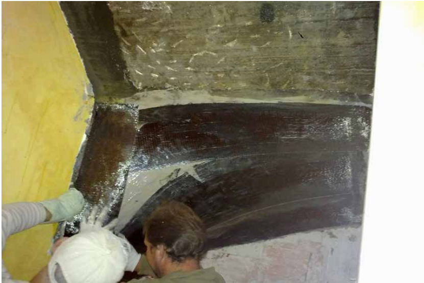
Structural reinforcement with carbon fibers
