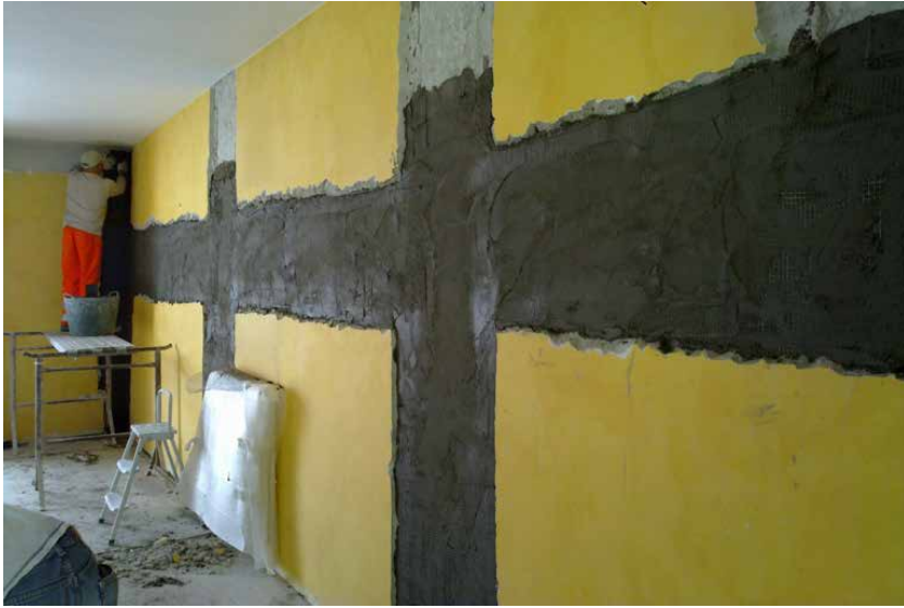
Structural reinforcement with fiber glass
