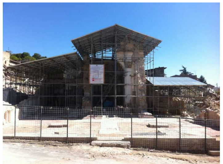
Special coverage and shoring in pipes and joints and Church of San Gregorio after shoring
