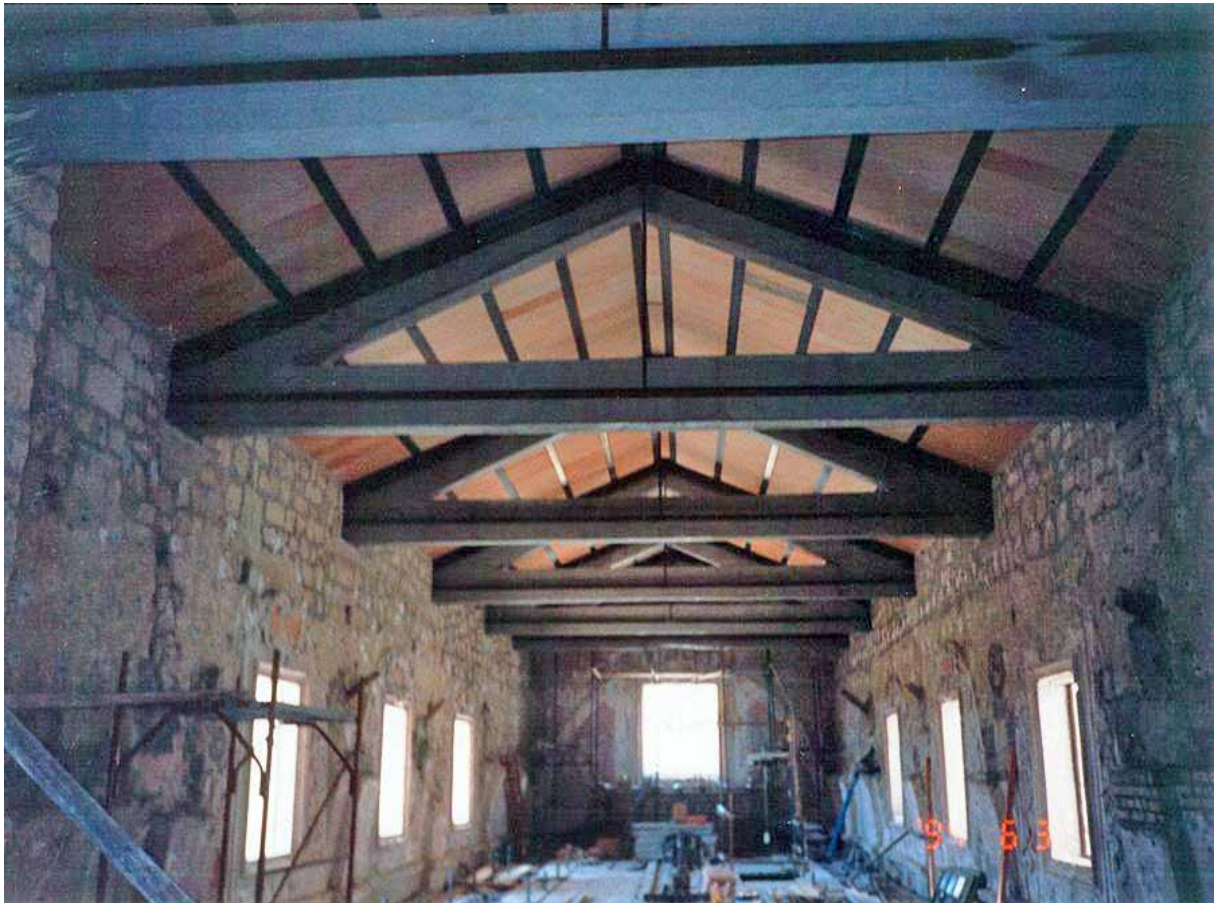
Particulars of the beams in CLS for the roof
