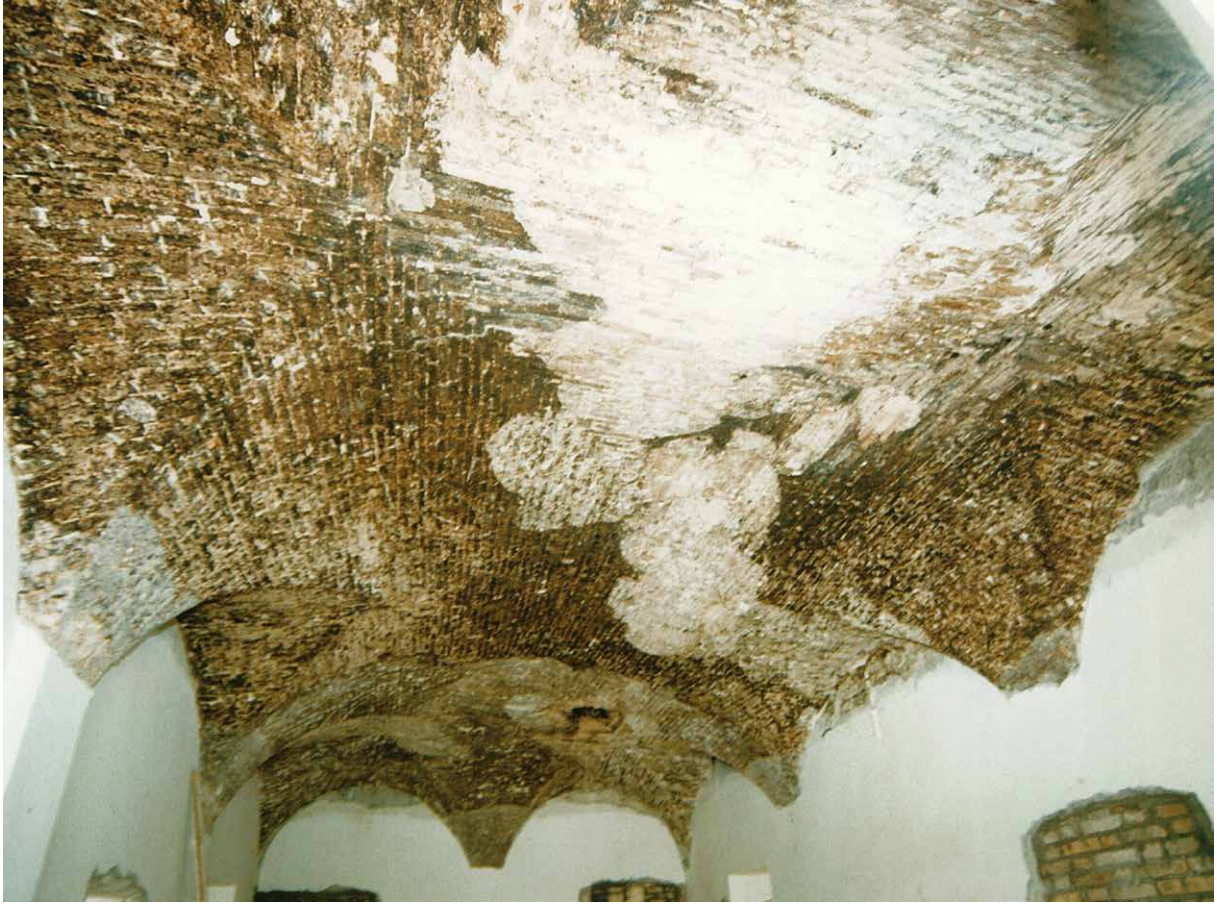
The vaults deteriorated before the restoration
