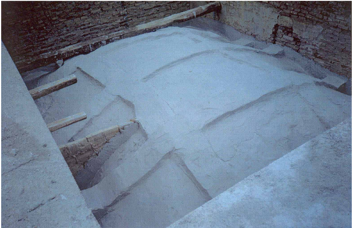
Vault after the consolidation
