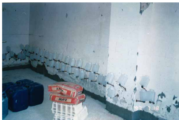
On the left execution of the chemical barrier against capillary rising moisture On the left the filling of the holes with special dehumidifying mortar
