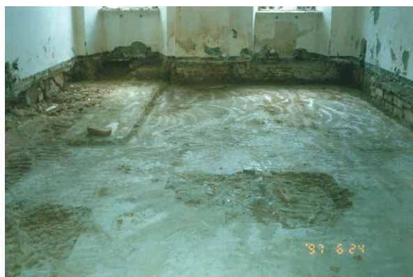
On the left the dismantling the floor for drainage – On the right laying of the nylon cloth and boards for drainage
