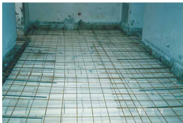
On the left installation of the iron for casting in CLSA – On the right verification tool with the percentage of humidity in the rooms
