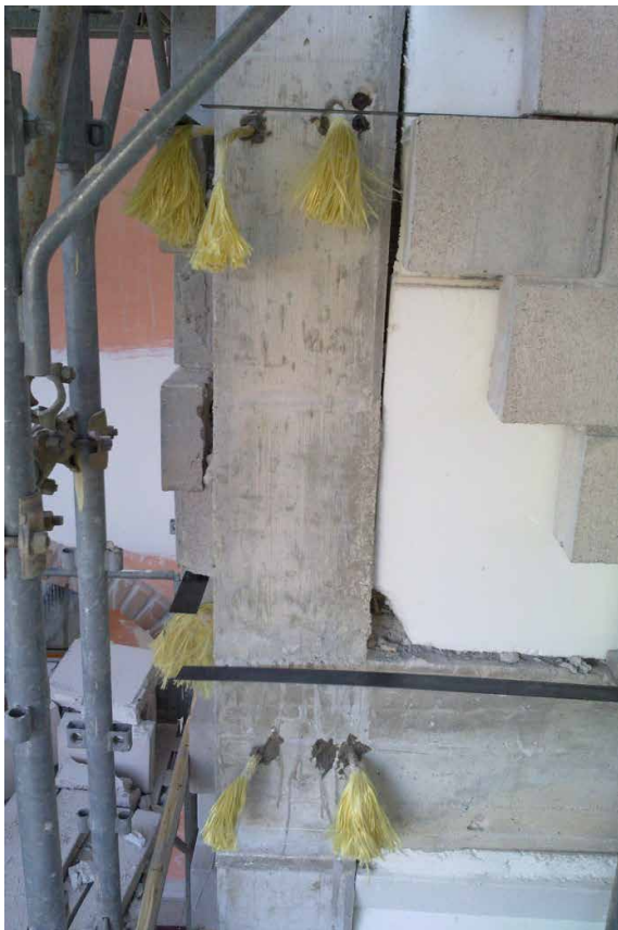
Restoration of the external curtain with aramedic fiber flakes and epoxy resins with the application of carbon foils
