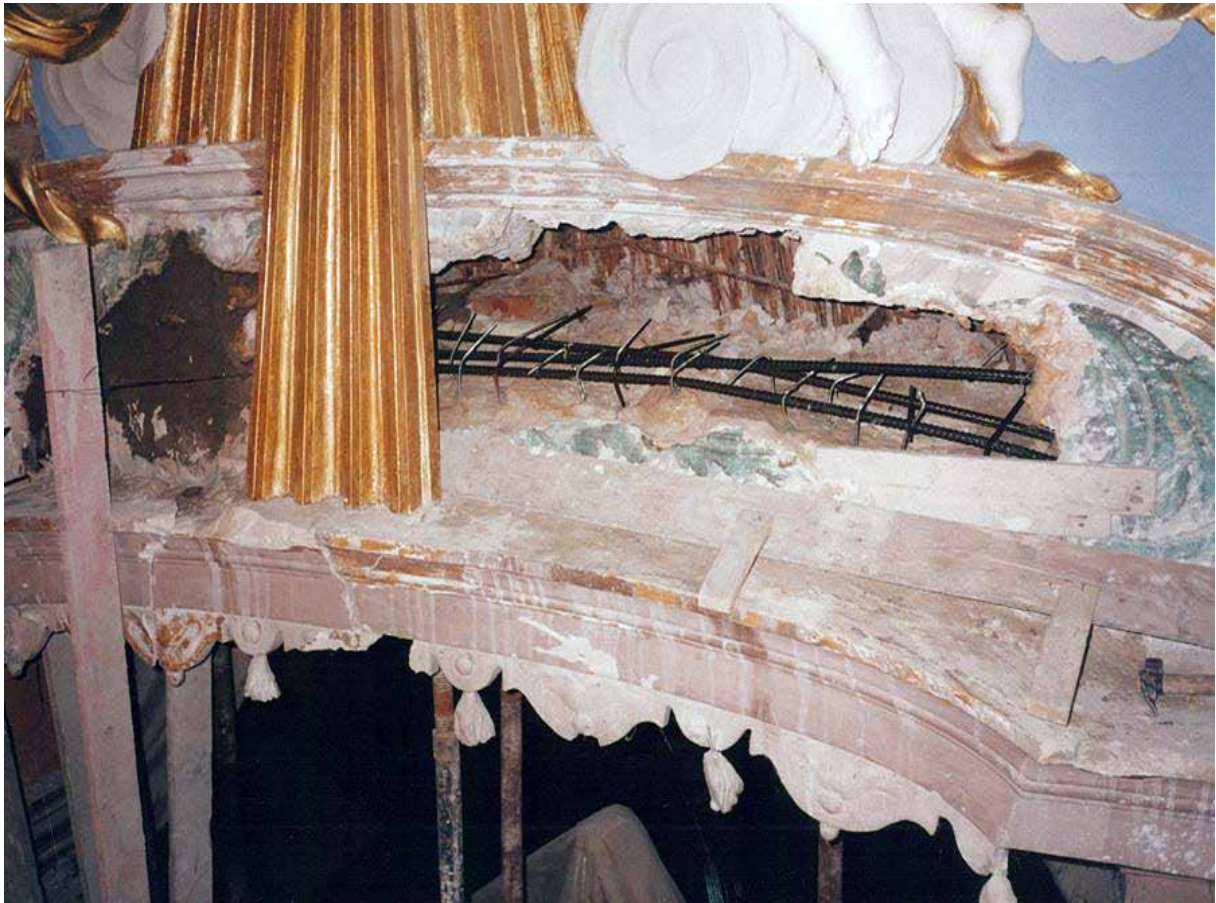
Particulars of the consolidation of the vault
