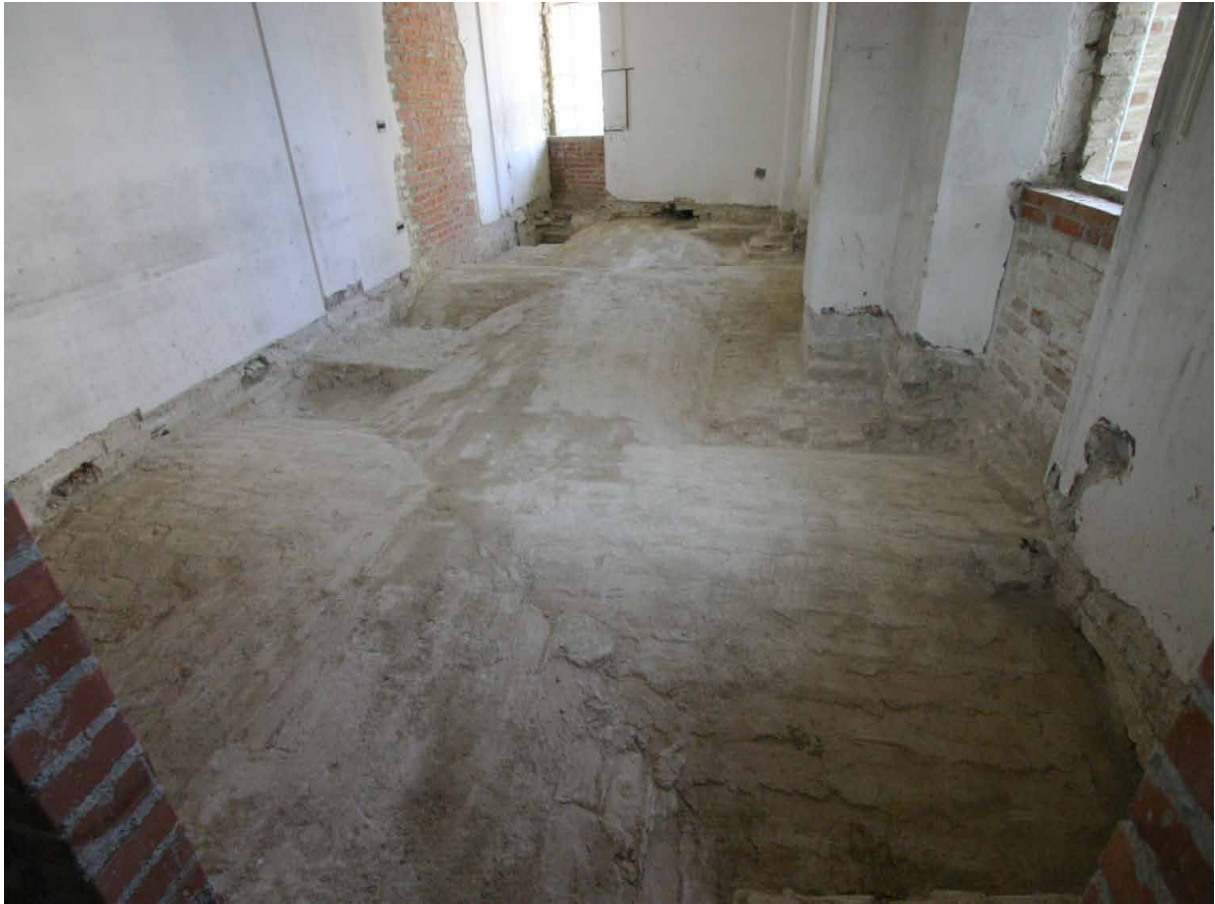
Consolidation of the vault: 1st working step: emptying the vault through the cleaning of the top surface
