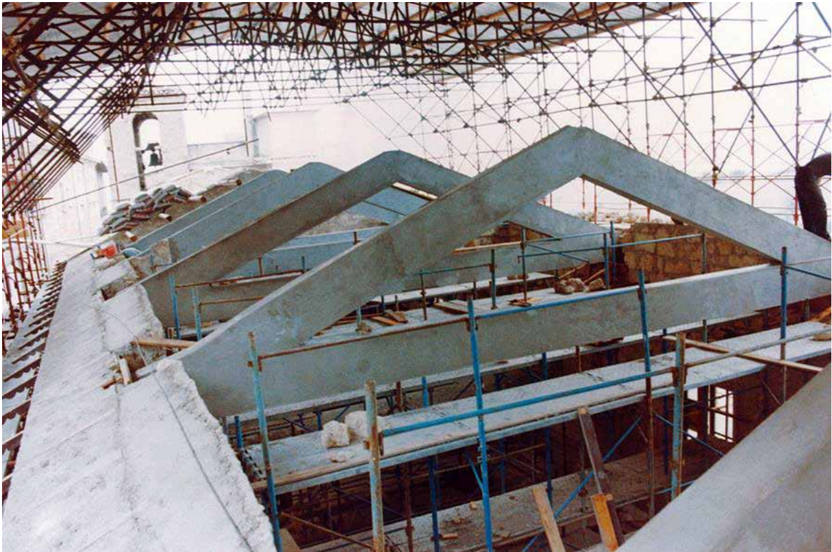
Particulars of the beams in CLS for the roof
