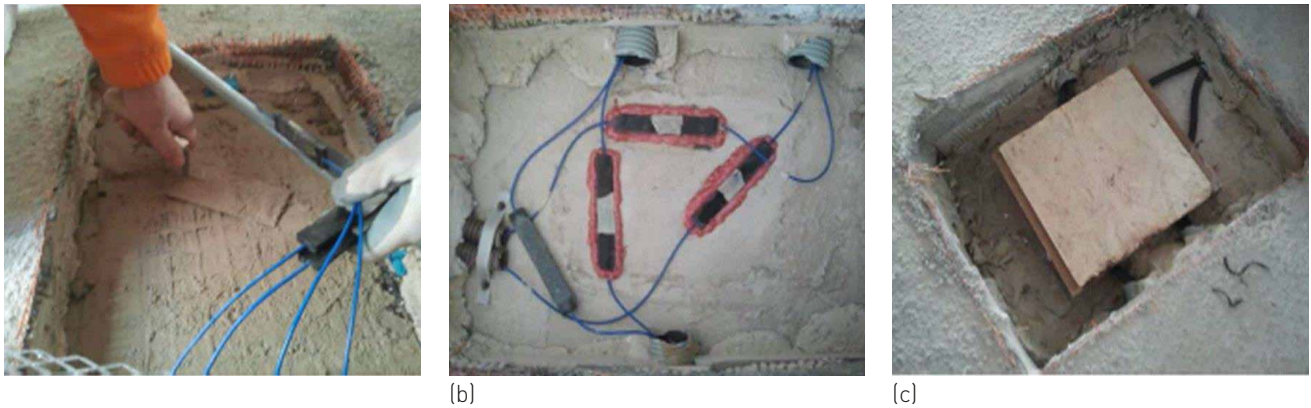
Figure 4: (a) Positioning of cable ducts and cables; (b) preparation of substrate and the gluing of sensors; (c) Protection of fiber and closures of boxes
