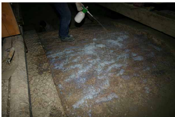
On the left particular deposit of a coat of retain grip to improve the adhesion of Malta On the right a particular of the under roof finished after consolidation
