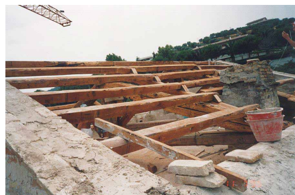
Total dismantling of the roof
