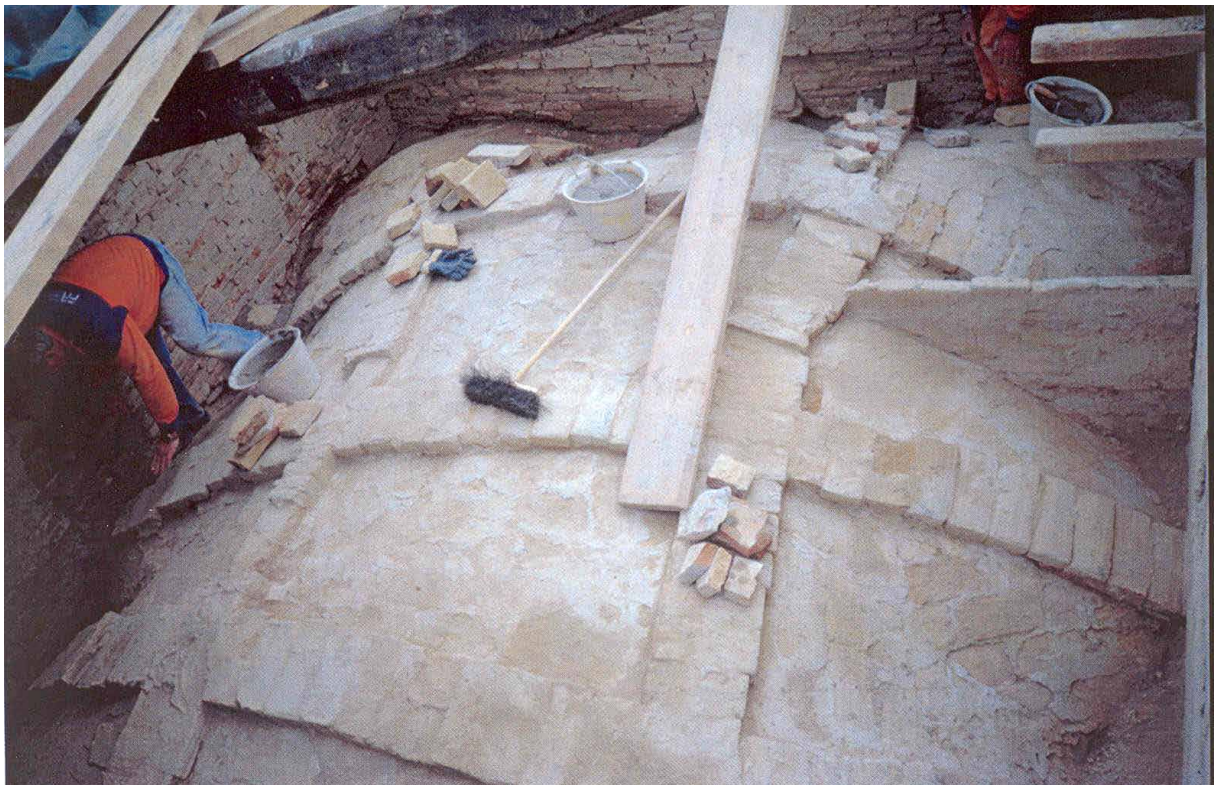
Restoration of the vault 2nd phase: renovation with the integration of the missing bricks and final cleaning
