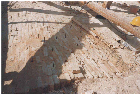
Specifics of the consolidation of the vaults of the attic
