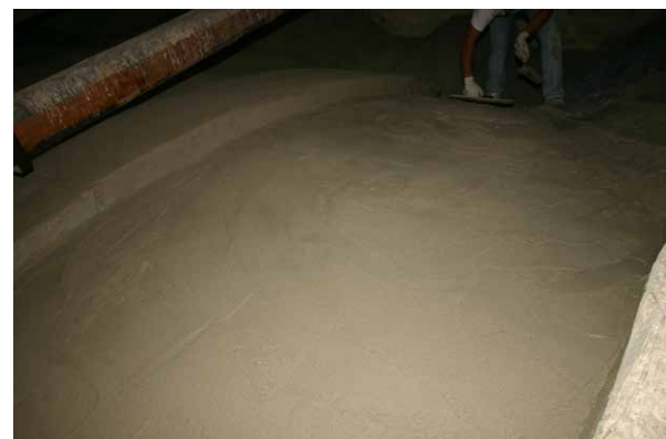
On the left particular deposit of a coat of retain grip to improve the adhesion of Malta On the right a particular of the under roof finished after consolidation
