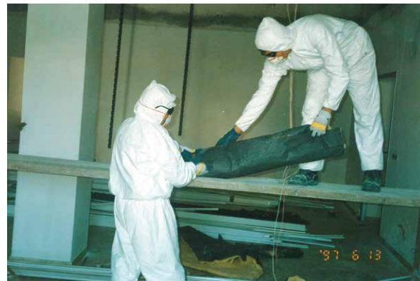
On the left rooms before restoration – On the right removal of mineral wool panels
