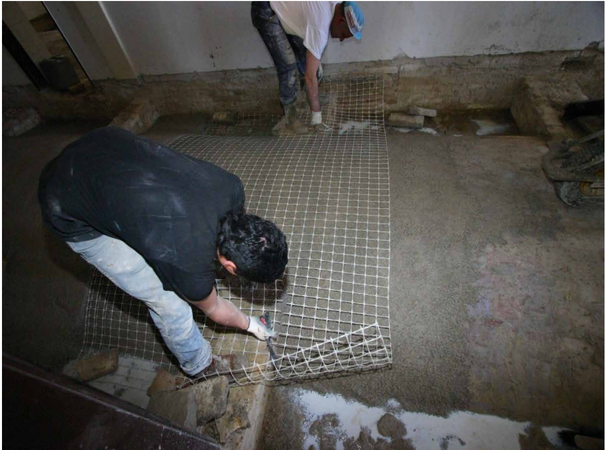
Consolidation of the vault: 3rd working step: installment of a wired biological polypropylene net
