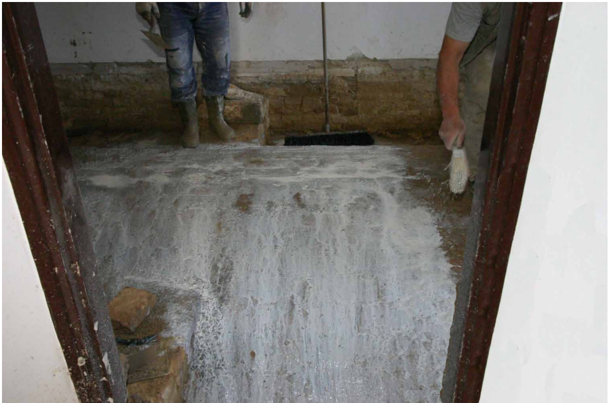
Consolidation of the vault: 2nd working step--the installation of a coat of retain grip to assure the perfect cohesion
