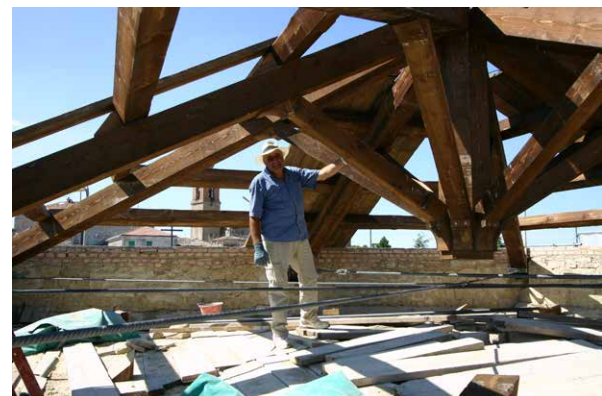
Particular replacement of the main cover frame
