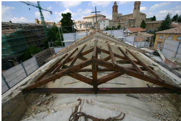
Particular replacement of the main cover frame
