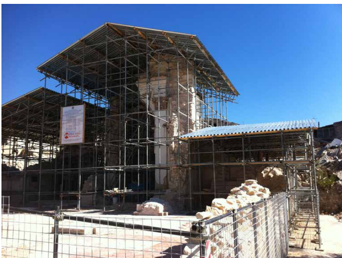
Special coverage and shoring in pipes and joints and Church of San Gregorio after shoring
